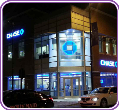
Downtown Skokie is celebrating a brand new Chase Bank branch at 7941 Lincoln Avenue, replacing the former Traeger Furs store with a two-story, state-of-the-art new facility.
